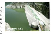
designed for PMF of 15540 m<sup>3</sup>/s and a drop of 220 m and an underground Power House containing four Turbine/Generator sets of 250 MW each, designed to operate with a head variation of 90 m. Project was commissioned in 2006-07 and all four machines of Tehri Power Station are under commercial operation.
